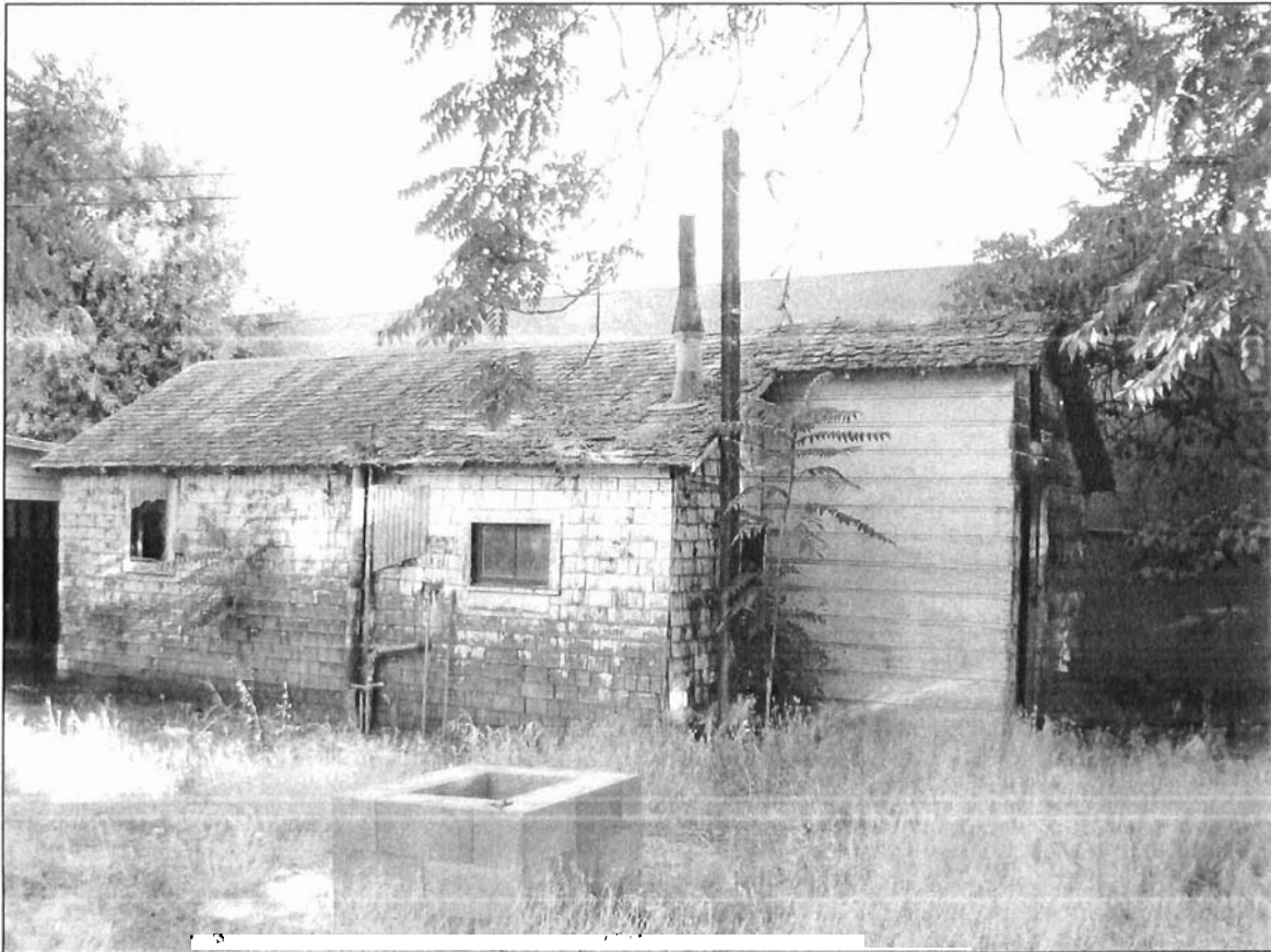
Plate 5. North elevation at 719 Pine Street.
