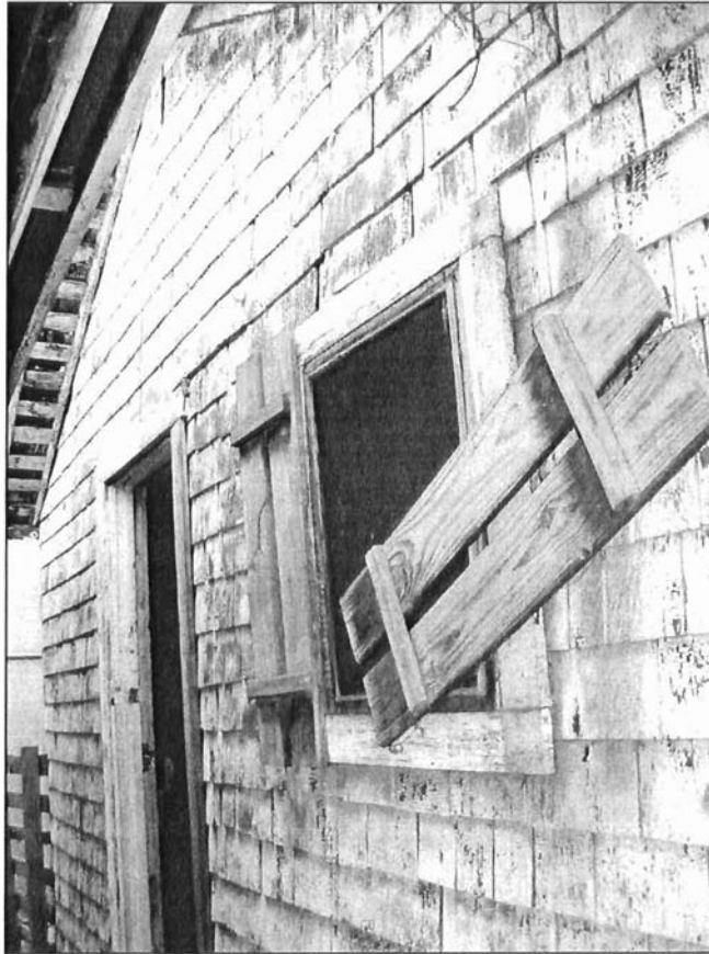
Plate 2. 719 Pine Street showing a portion of the east façade.
