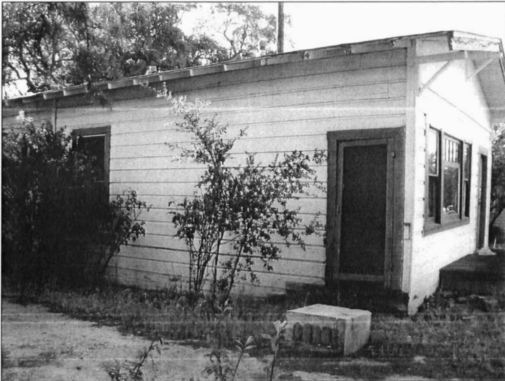
Plate 7. Eastern end of the south elevation at 721 Pine Street.
