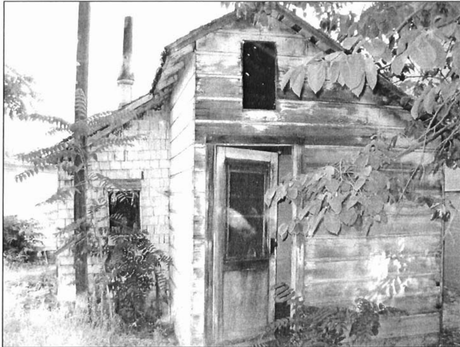
Plate 4. West elevation at 719 Pine Street.
