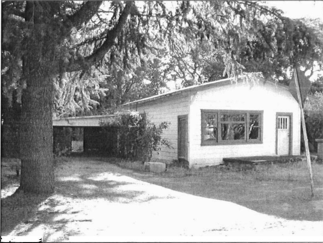
Plate 6. East façade at 721 Pine Street showing carport on south end
