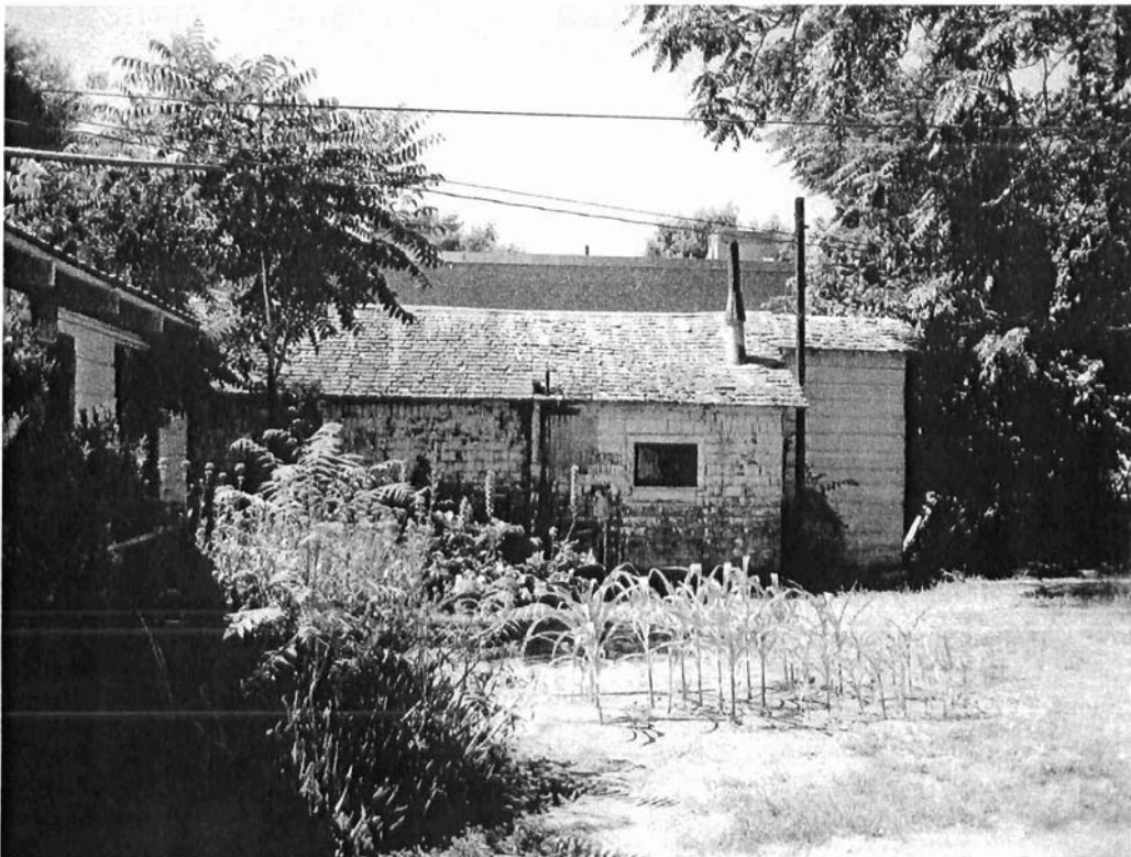
FACING SOUTH AT 721 PINE CONDEMNED RESIDENCE
